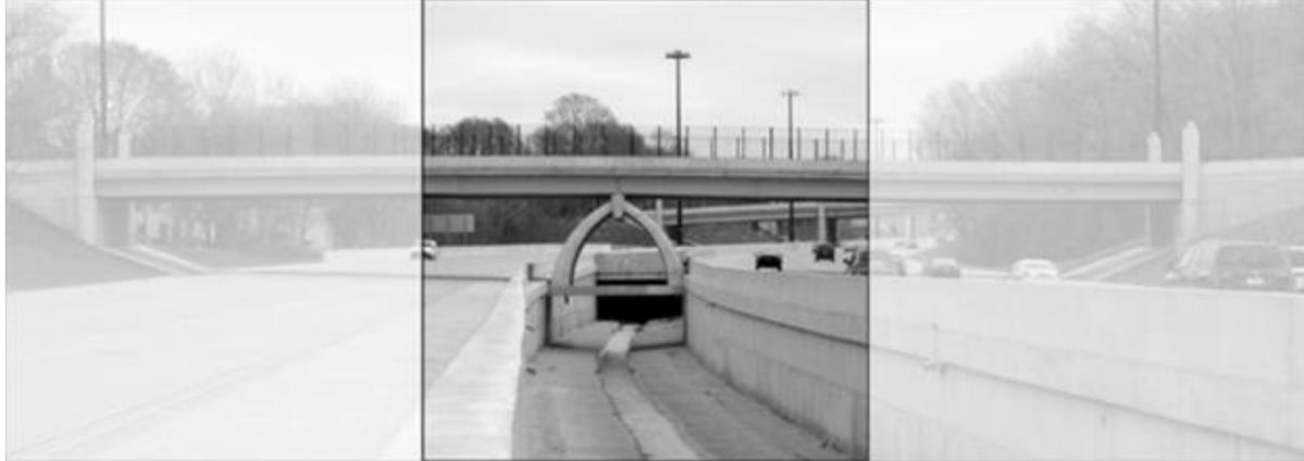
*Figure 6: Arch pier allows for pier construction without impacting the waterway below*
