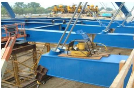
*Figure 8: Redundant cable strands*
